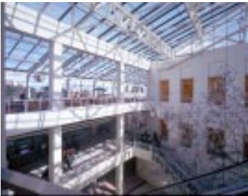
The light fixtures in this atrium are controlled by photosensors.
